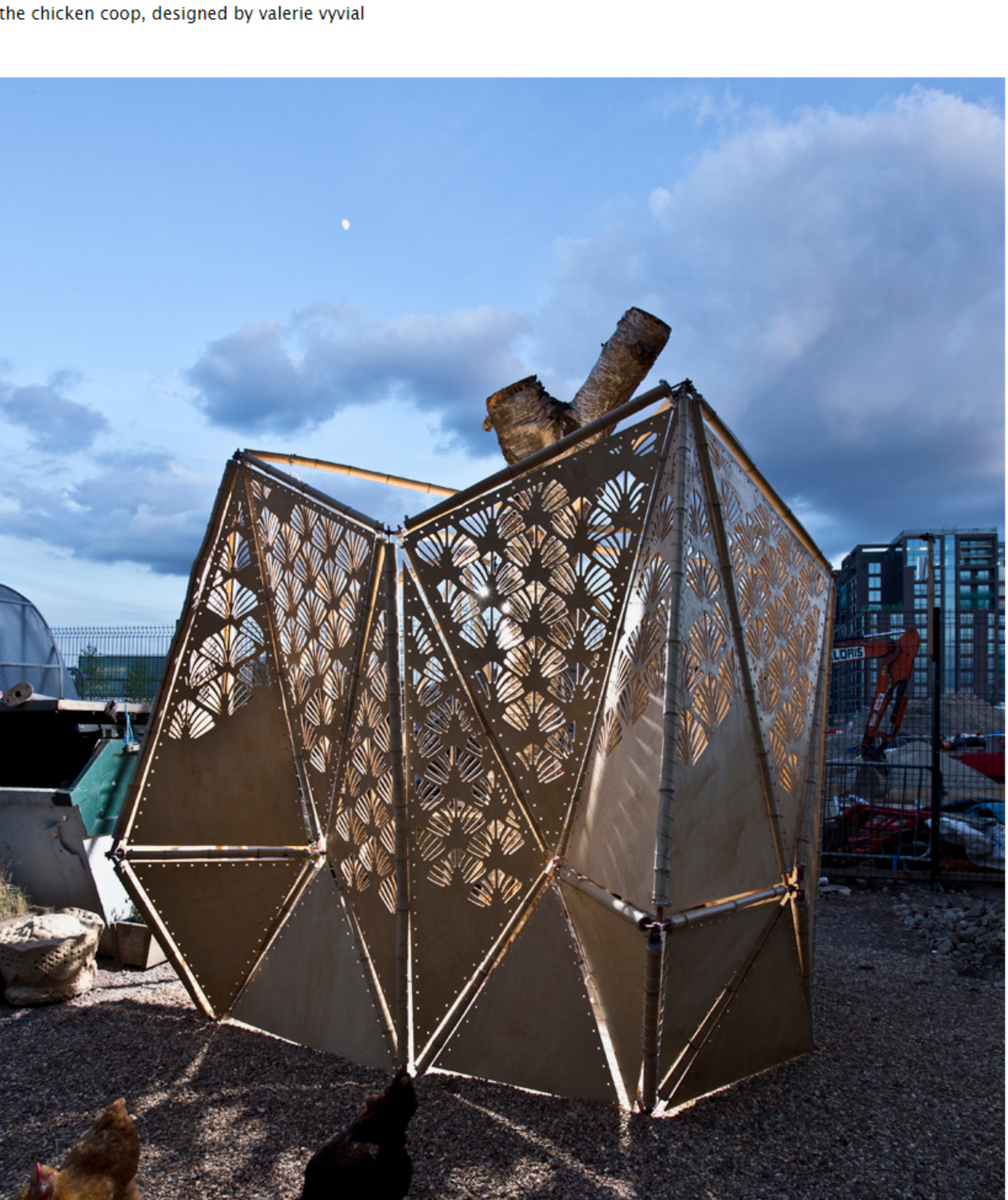
the primary structure is bamboo joined by steel fixings
