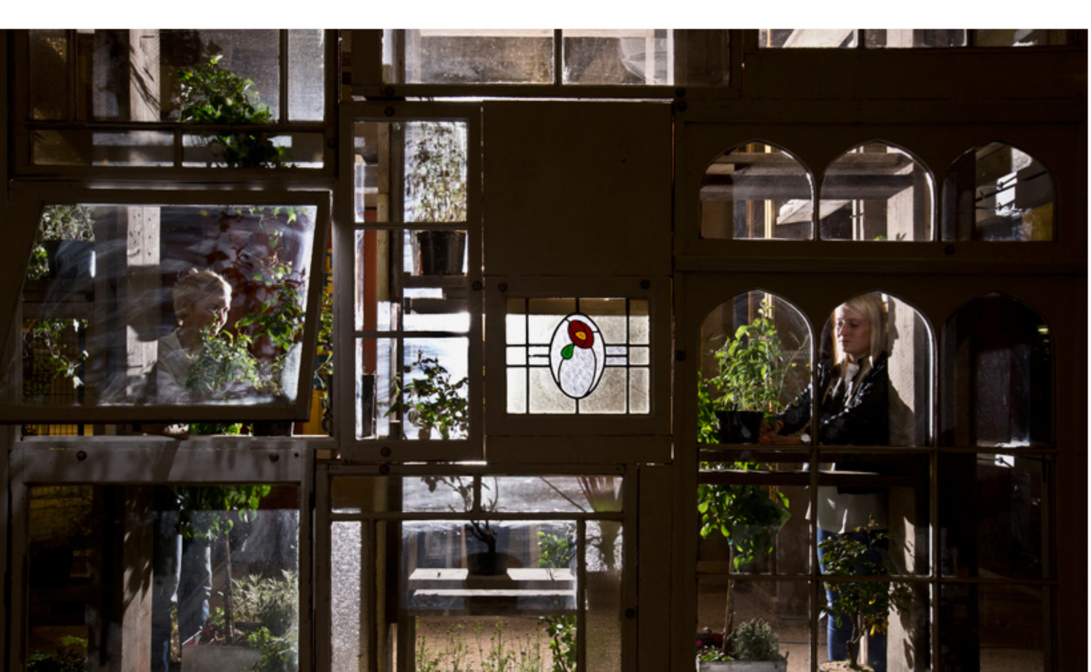
the reclaimed windows are used to create a greenhouse effect
